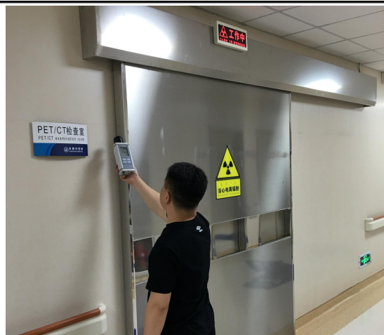
PETCT 机房防护门外检测
